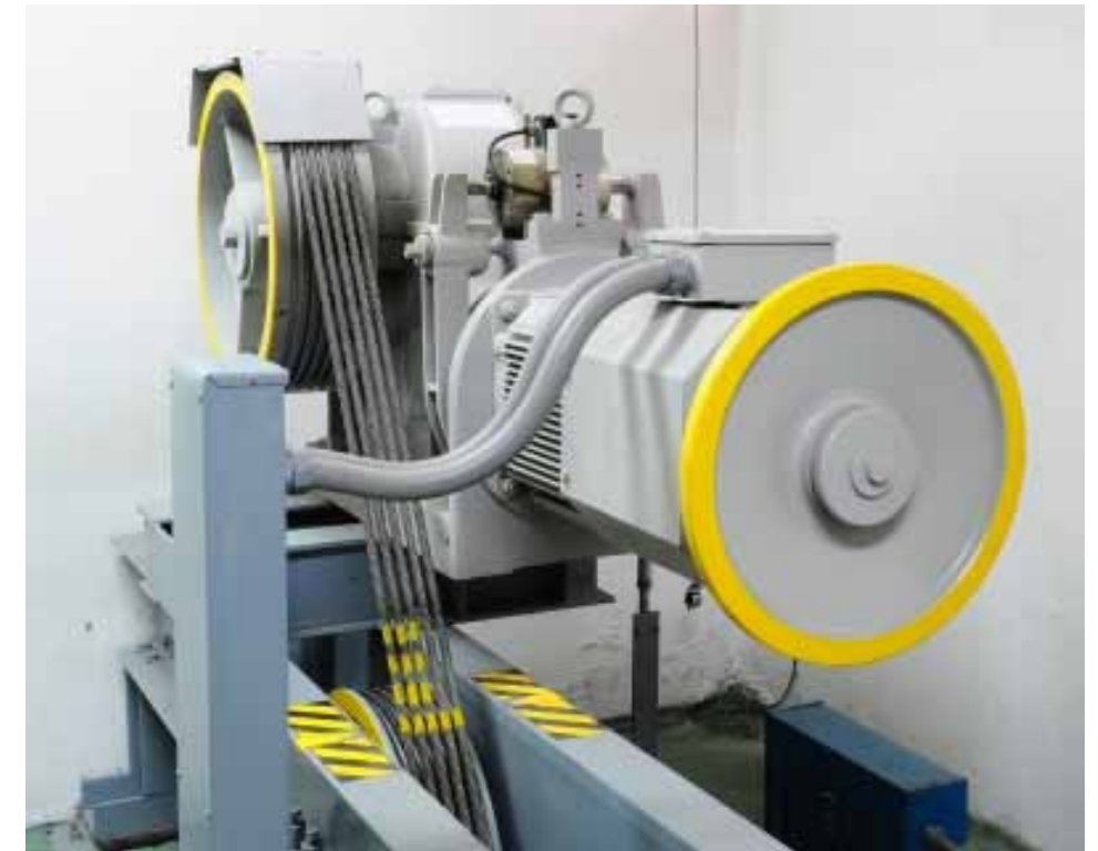
MOTOR DRIVEN ELEVATOR IN THE ENGINE ROOM COURTESY OF TWOBEE - FREEDIGITALPHOTOS.NET
