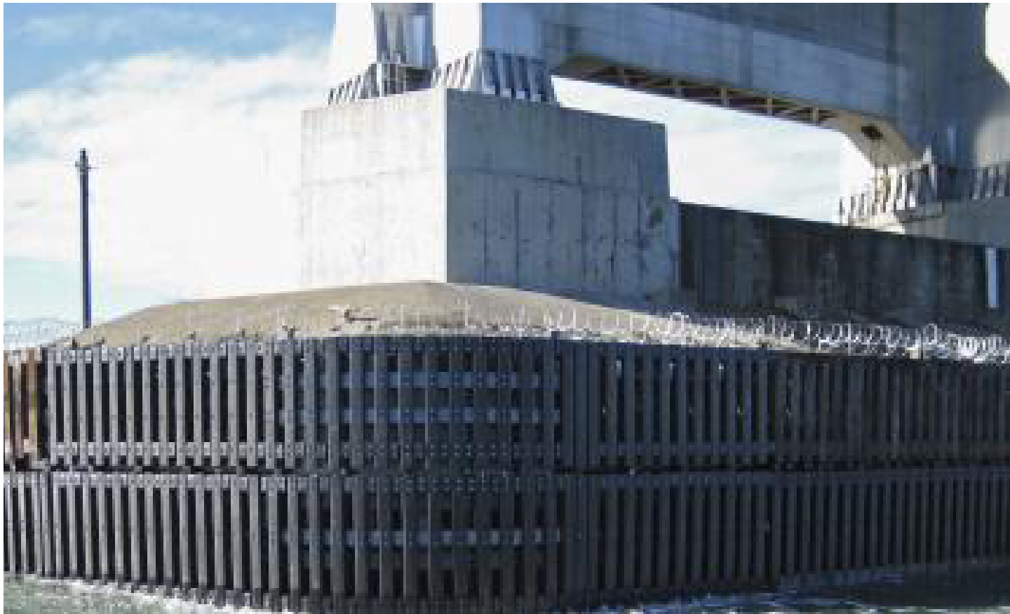
FIGURE 2: SEATIMBER'S PLASTIC MATRIX IS REINFORCED WITH GLASS FIBER TO WITHSTAND THE WEAR AND TEAR OF MARINE ENVIRONMENTS FOR DECADES, EVEN ABSORBING THE IMPACT OF LARGE OCEAN-GOING VESSELS
