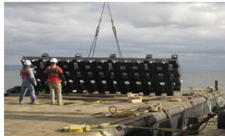
FIGURE 1: INSTALLING THE SEATIMBER’S PLASTIC MATRIX
